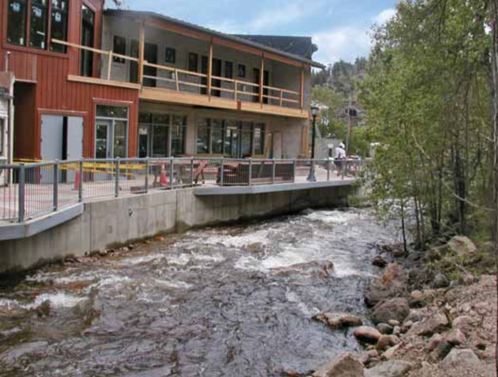
For the most part, site-poured concrete retaining walls were left plain to maintain year-to-year consistency. A form liner has given the surface some texture. (Photo courtesy Heath Construction)
